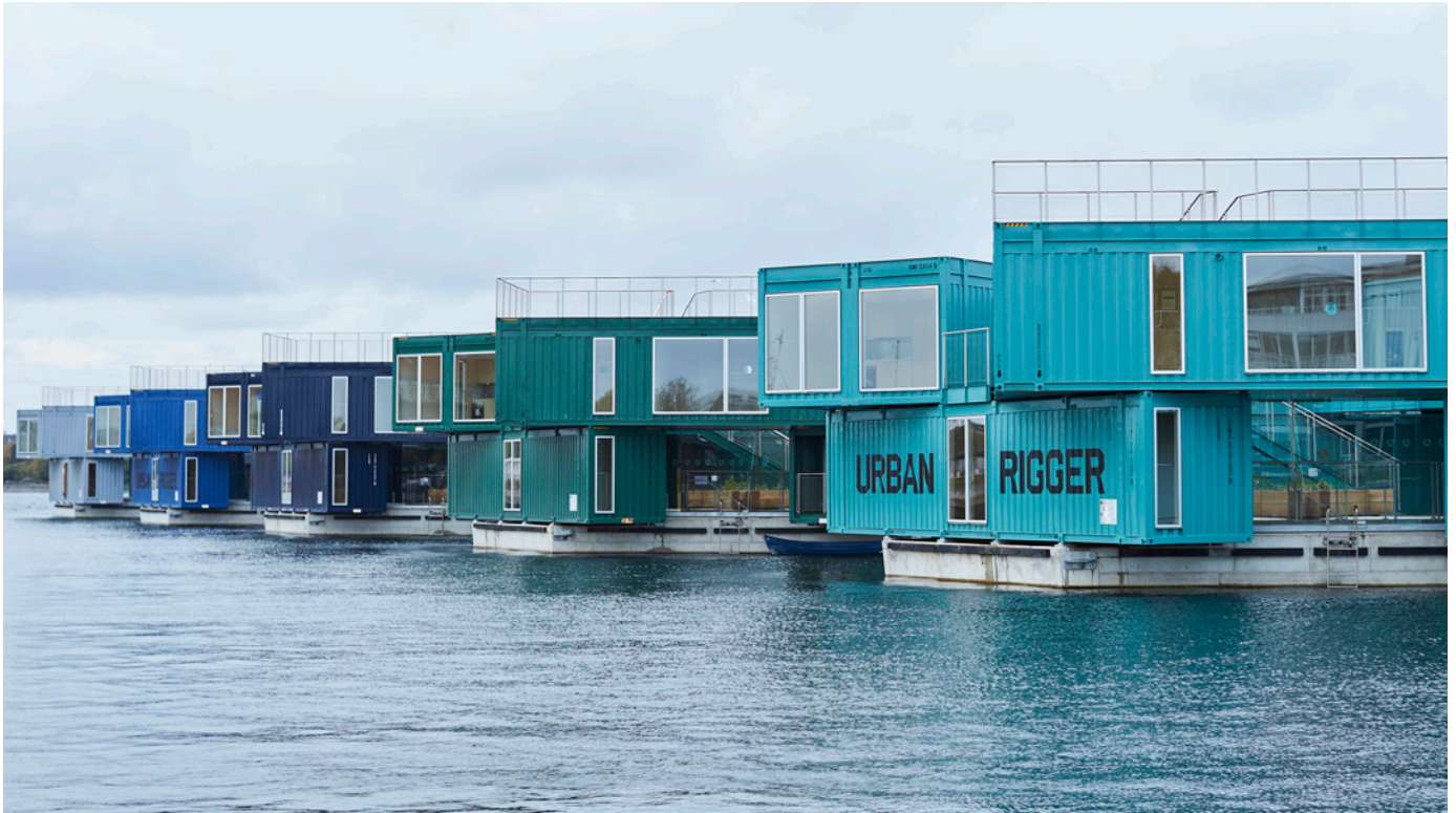
Urban Rigger floating structures in Copenhagen. Credit: Urban Rigger
