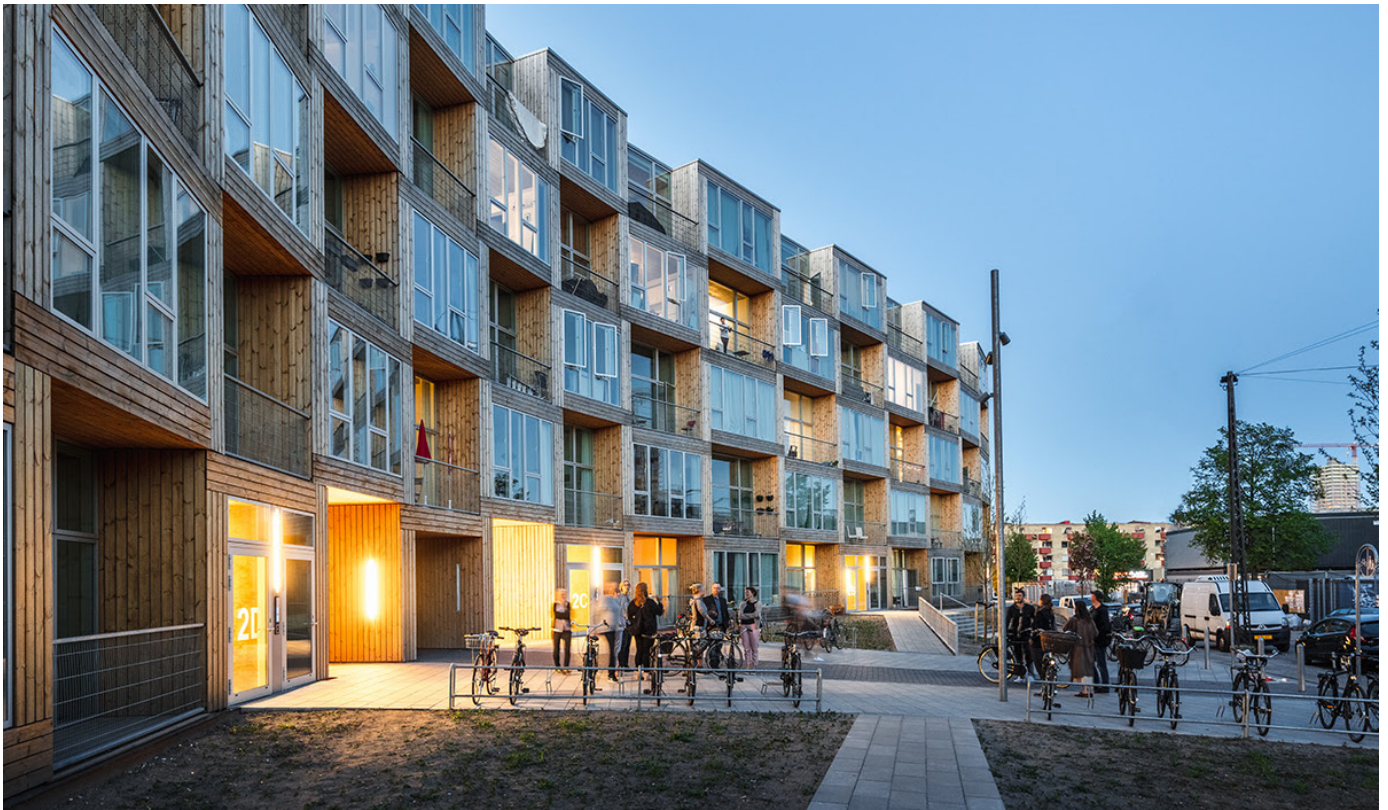
Dortheavej Residence with cycle parking. Credit: Bjarke Ingels Group
